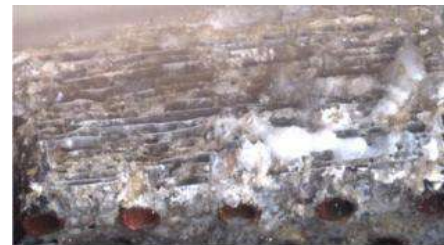
Unprotected coil after 4000 hours acid spray test
