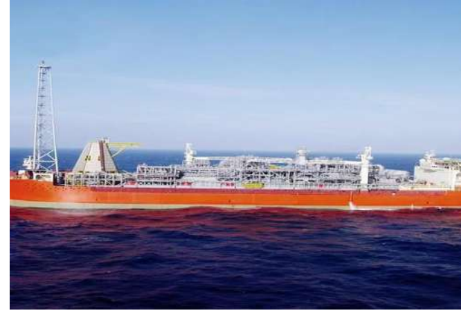
Offshore Texaco Captain Production Platform
