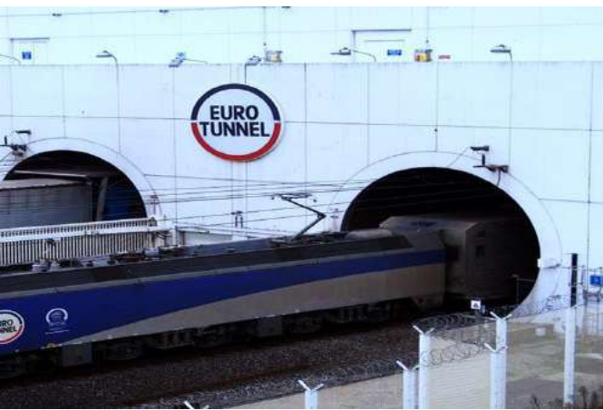
Construction Channel Tunnel France to UK
