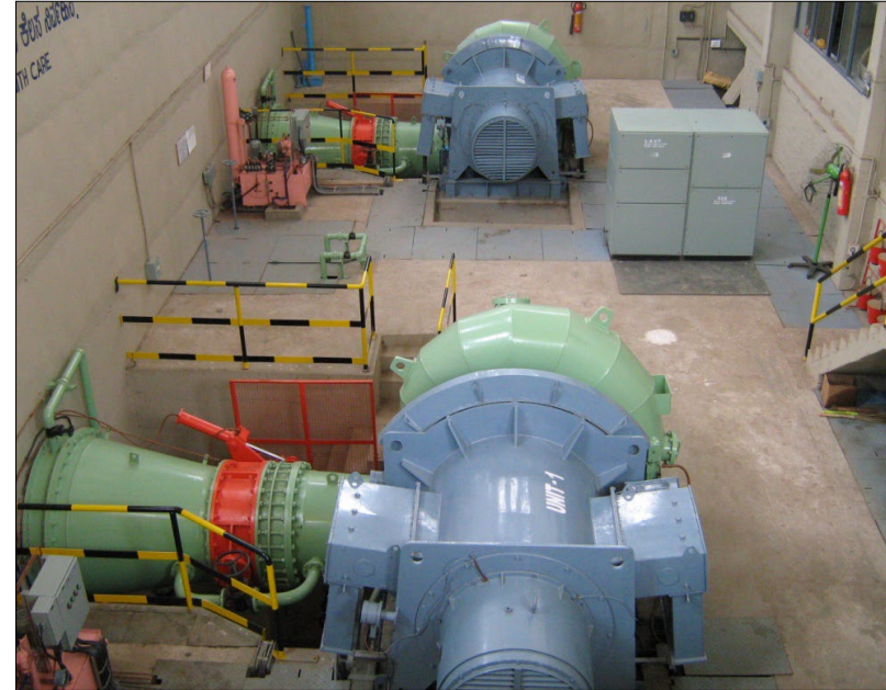
Nugu -II HEP 2 x 750 kW Horizontal Francis Runner Dia. 780mm, Head 28 m
