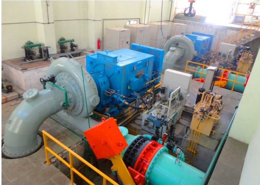
Sechi HEP 2 x 2250kW Horizontal Francis Runner Dia. 660mm, Head 134.85 m
